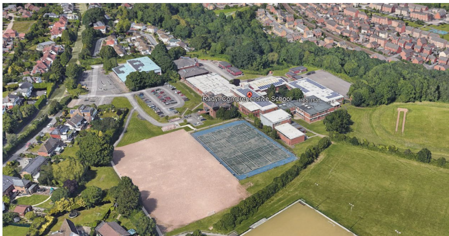
Fig. 1 – View from the South West across the School Campus
